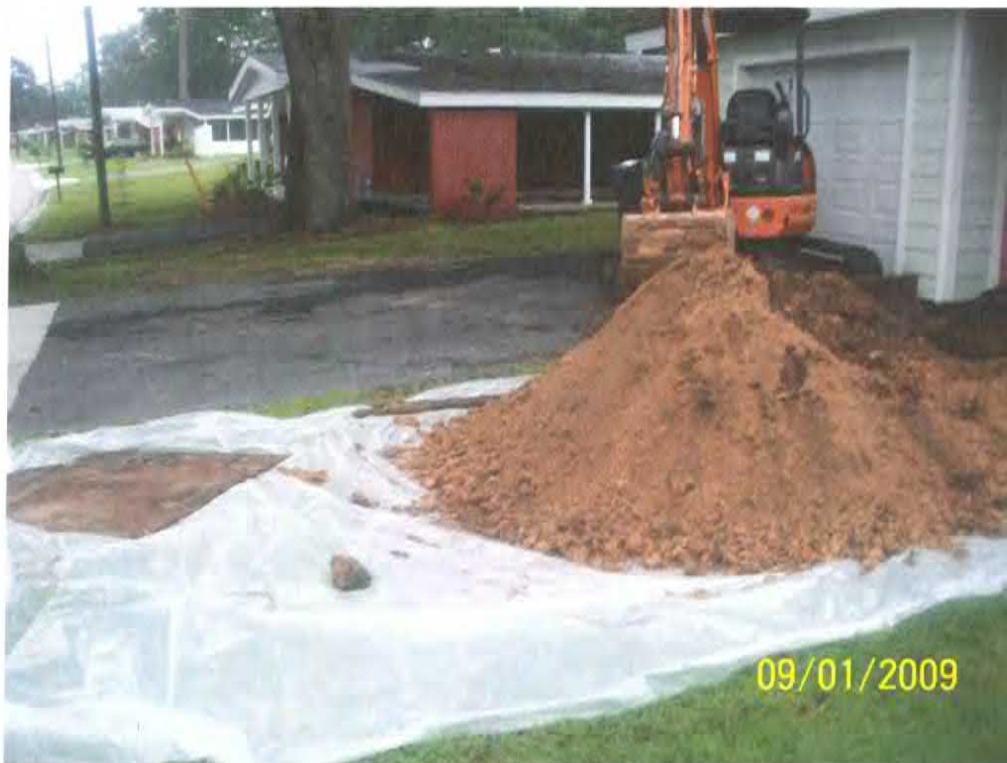
Picture 2: UST 1250Dove removal in progress.
